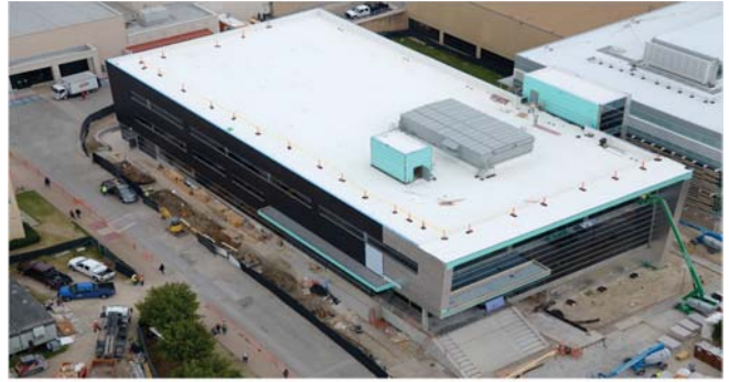
J E Dunn Construction UTD Student Services Building Photo #161102052 Date: 11/02/16 Lat/Lon: 32.980236 -96.748432 Order No: 59707 Aerial Photography, Inc. 954.988.0484
